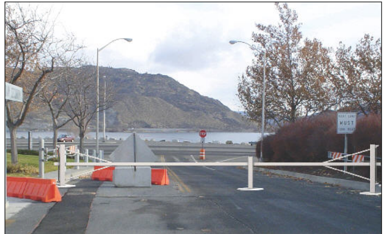
Combination Swing Arm Gate with removable center superpost.
